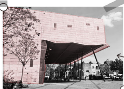
The new library is located on the west side of the building.
