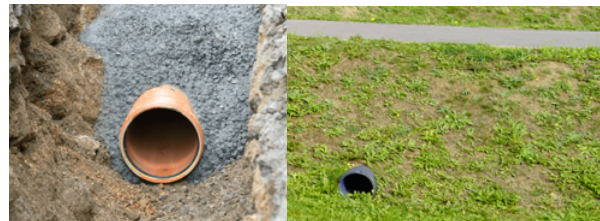
Pre-embedded permeable pipe for road re-construction
