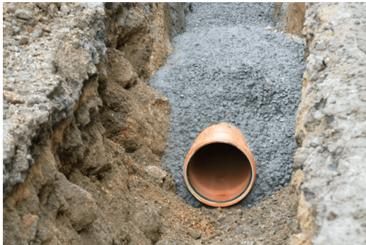
Pre-embedded drainage pipes
