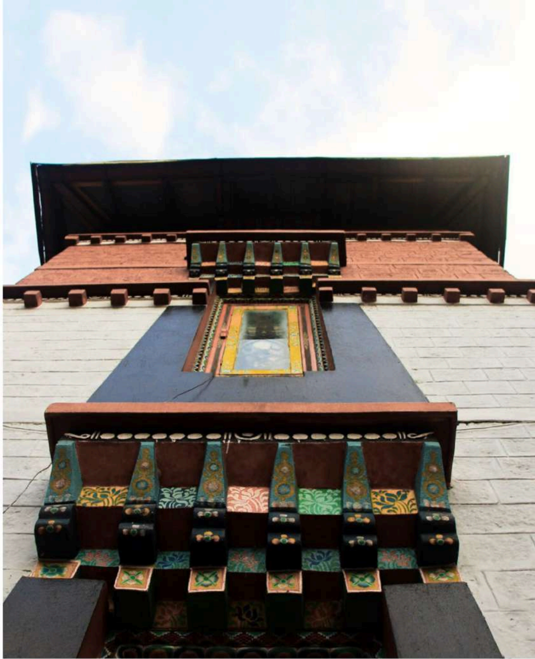
fig 32: Traditional architecture openings in NIT
