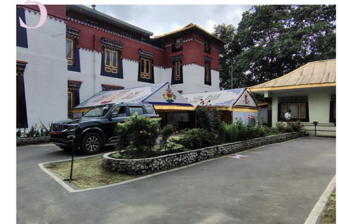
courtyard currently used for parking
