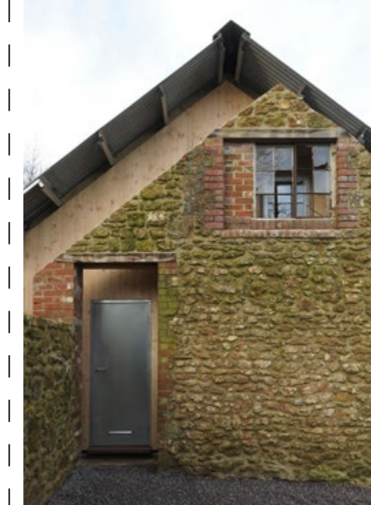
Architects' Archive , Hugh Strange(2014)
