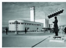
Ankara Opera House, designed by Şevki Balmumcu (1933-34) and renovated by Paul Bonatz (1946-47).
