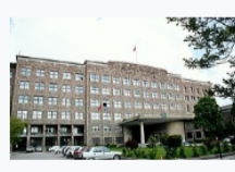
The Faculty of Languages, History and Geography building (1937) of Ankara University was designed by Bruno Taut.
