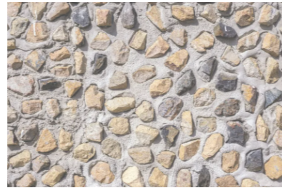
Mixed stone with recycled asphalt aggregate
