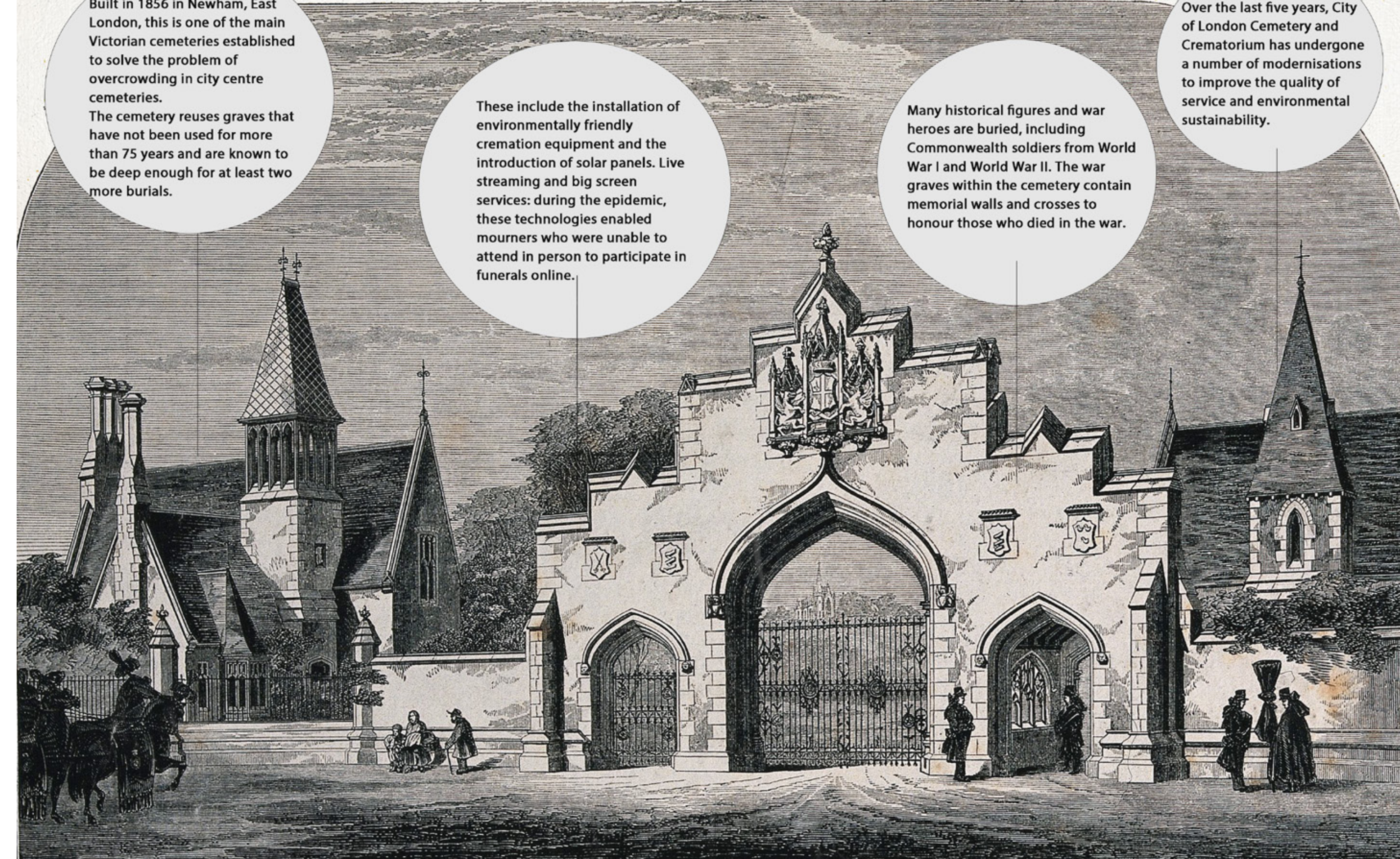
ENTRANCE GATEWAY, CITY OF LONDON CEMETERY.—MR. WILLIAM HAYWOOD, ARCHITECT.
