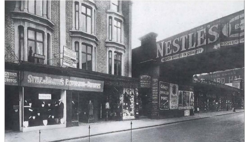
Style & Mantle's and Baker & Norman occupied 107-109 and 113 Rye Lane in the 1920s. The Tower Cinema advertisement shows that a Charlie Chaplin film was being shown. Between the railway lines Holdron's had a shop. (John D, 2010, 43)
