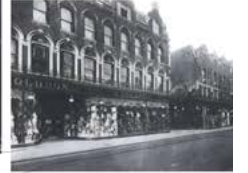
1920, 135~147 Rye Lane, Holdron's Main Building
