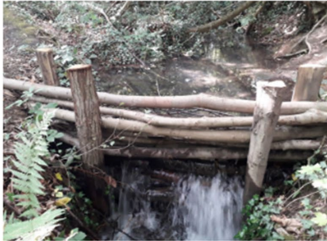
A leaky dam: one example of natural flood management
