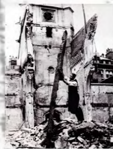
New York Bureau: "Because many of the City's churches remain filled with debris and buried treasures as municipal demolition workers must concentrate on business and residential bombed areas, the Revd Dr Frederick C Oliver, of the church of St Dunstan-in-
